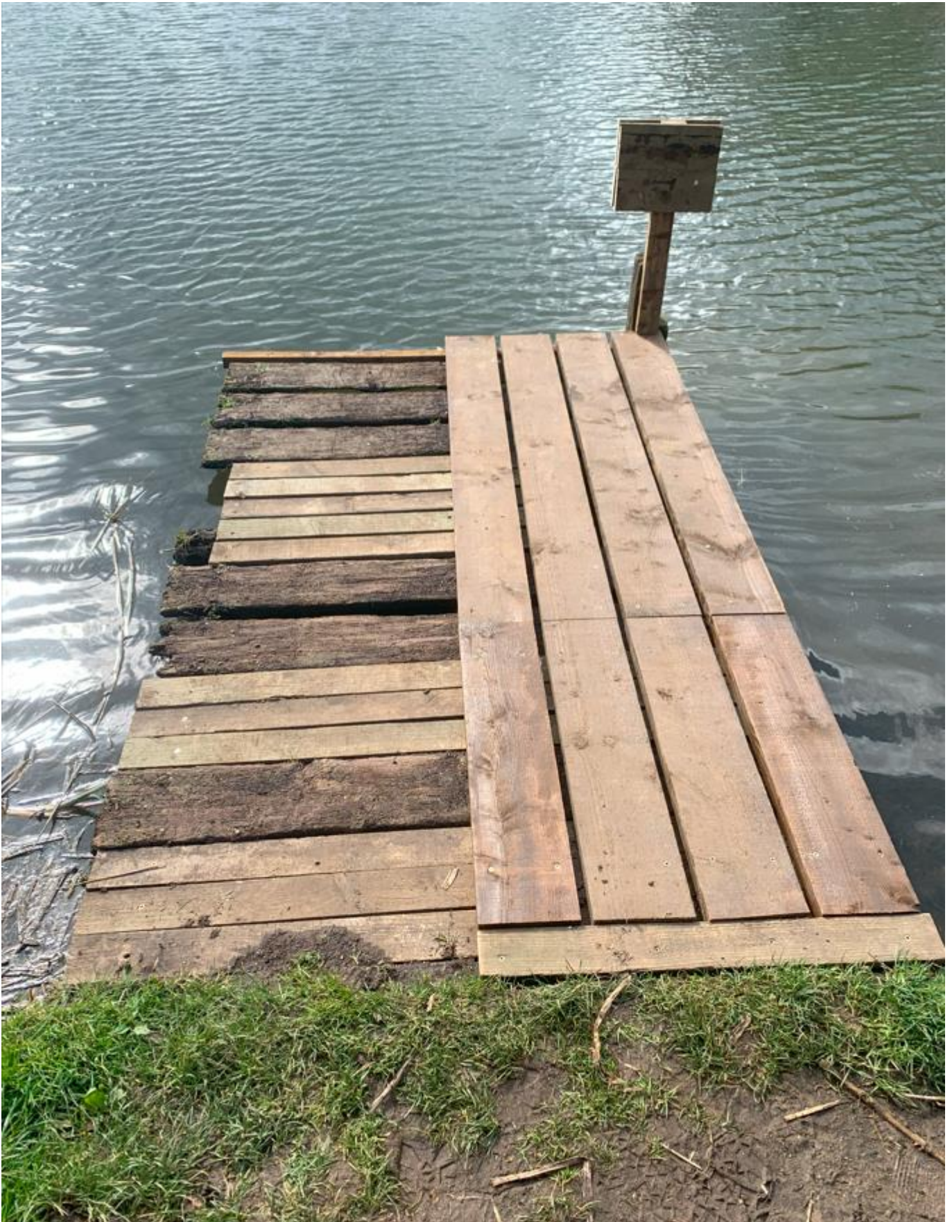
13. Picture of current canoe portage after temporary repair.
